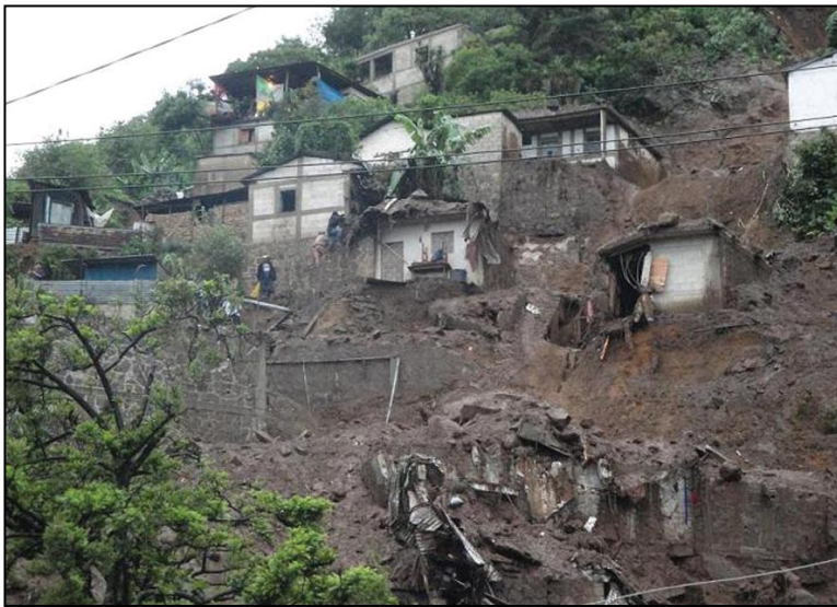
One of the 22 mudslide areas in San Antonio Palopo. This was an area filled with homes prior to the storm.
